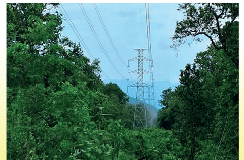
BHARATPUR-BARDAGHAT TRANSMISSION AFTER 13 YEARS
