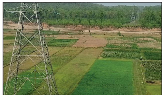
BHARATPUR-BARDAGHAT TRANSMISSION : After 13 Years
